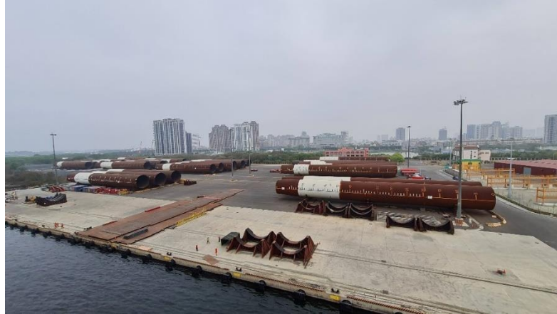
Figure 8-4: Monopile storing at Ports on cradles for OSW in Yunlin, Taiwan [13]
