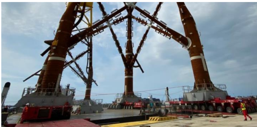
Figure 8-9: Discharge with 1 x SPMT under each leg
