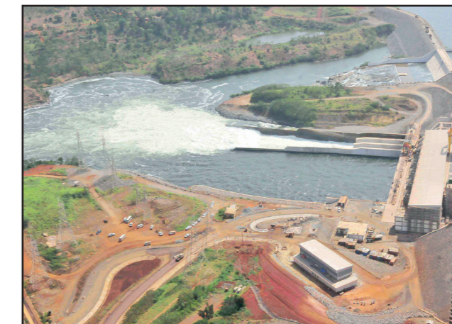
Bujagali Hydroelectric Power Station partly owned by Scatec (a Norwegian company) with investment from Norway's development financing agency, Norfund
