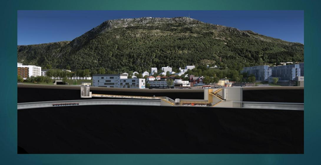
Construction stage4: 3 km tunnel for train with tunnel running parallell for bicycling and walking.
